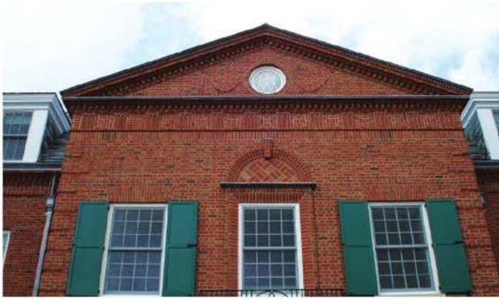
Also pictured on page 20, the Hotchkiss School dormitory demonstrates the versatility of load-bearing concrete masonry units (CMUs). They support the structure and form the backup for the brick veneer.
